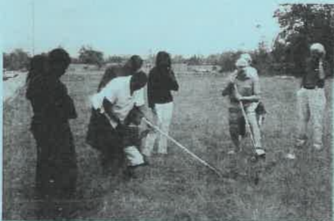
Gbenga and Lanre Balogun and family break ground on the 25th Habitat home July 16th on Summit Street.
