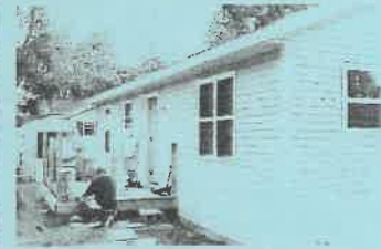
Juna Koonst home currently under construction at High and Perry Streets
